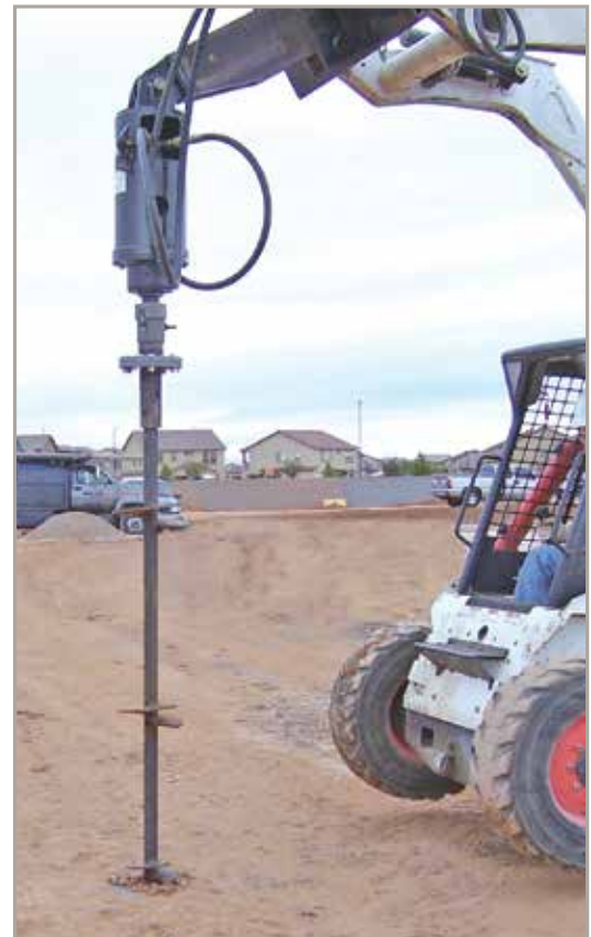
Typical MB Brace Badger Installation
