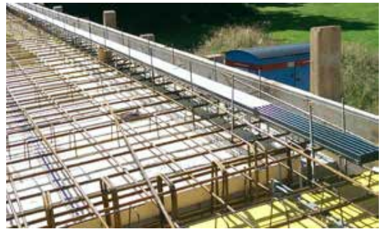
Installation with trench drain elevation
