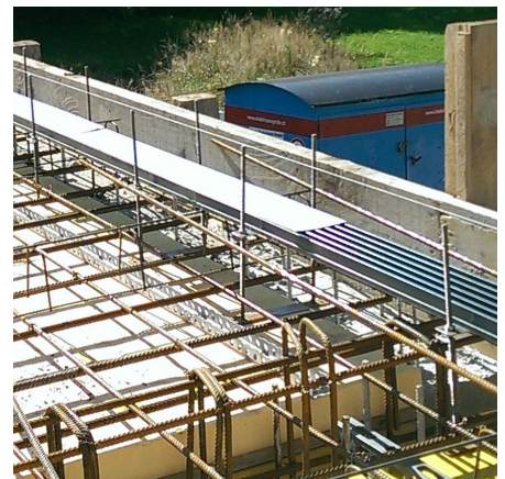
Installation with elevation bracket
